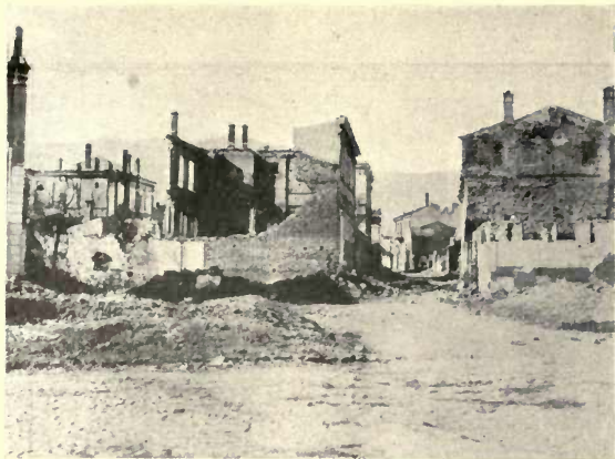
MONASTIR. EFFECT OF THE FIRE CAUSED BY INCENDIARY SHELLS.
