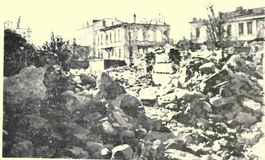
MONASTIR. EFFECT OF THE FIRE CAUSED BY INCENDIARY SHELLS.
