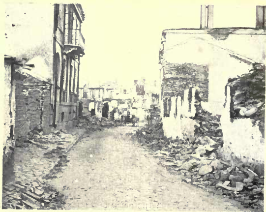
MONASTIR. HOUSES DESTROYED BY INCENDIARY SHELLS.
